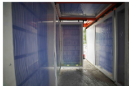
Completed Cold Tube
